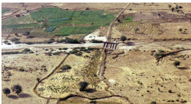
Aerial view of a water-spreading weir, Chad (Heinz Bender).
