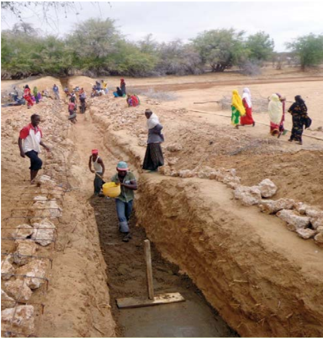
Excavation process (from IUCN archive).
